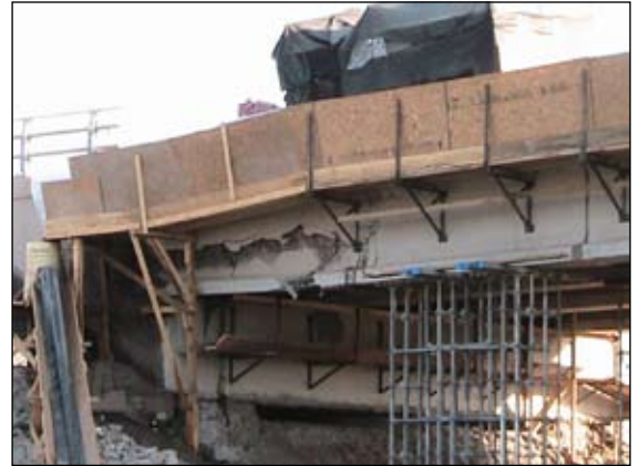
Serious earthquake damage.
