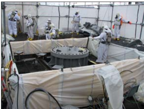
A Hanford Site crew installs a plug into the hole that AK Services cut.
