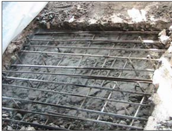
The Aqua Cutter proved ideal to remove the concrete above the damaged beams.
